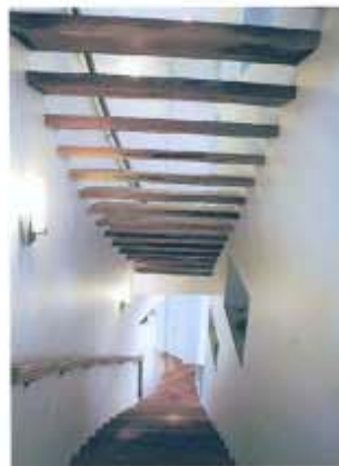
▲ An open staircase sucks warm air up to the third floor, where it is blown out a lowered window in the attic by a 4-foot-wide fan.
