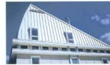
◀ The roof is pitched at 30 degrees so sunlight can penetrate its solar panels at a perpendicular angle, thus maximizing the amount of energy generated. Says Bingler: 'Even though it looks arbitrary, it's not arbitrary. Virtually everything in this house is here for a reason.'
