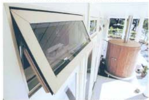
◀ A 1,200-gallon wooden cistern, lined with fiberglass, sits on the side porch to collect rainwater, which is used to flush toilets, wash cars and water plants.
